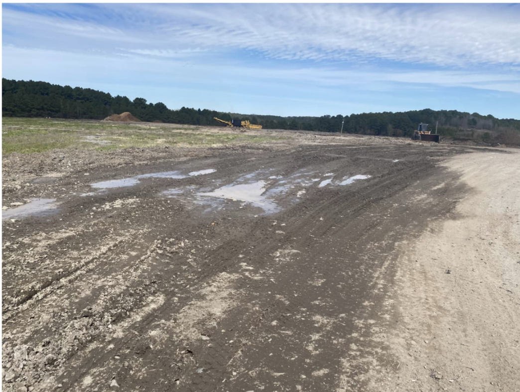
Standing near SW corner of Compost area / Looking NE
