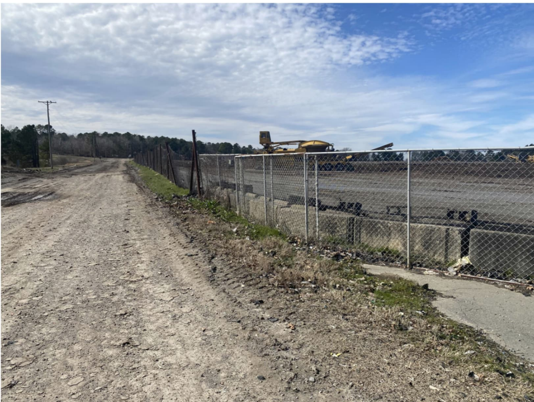
Standing at SE corner of Compost area / Looking west
